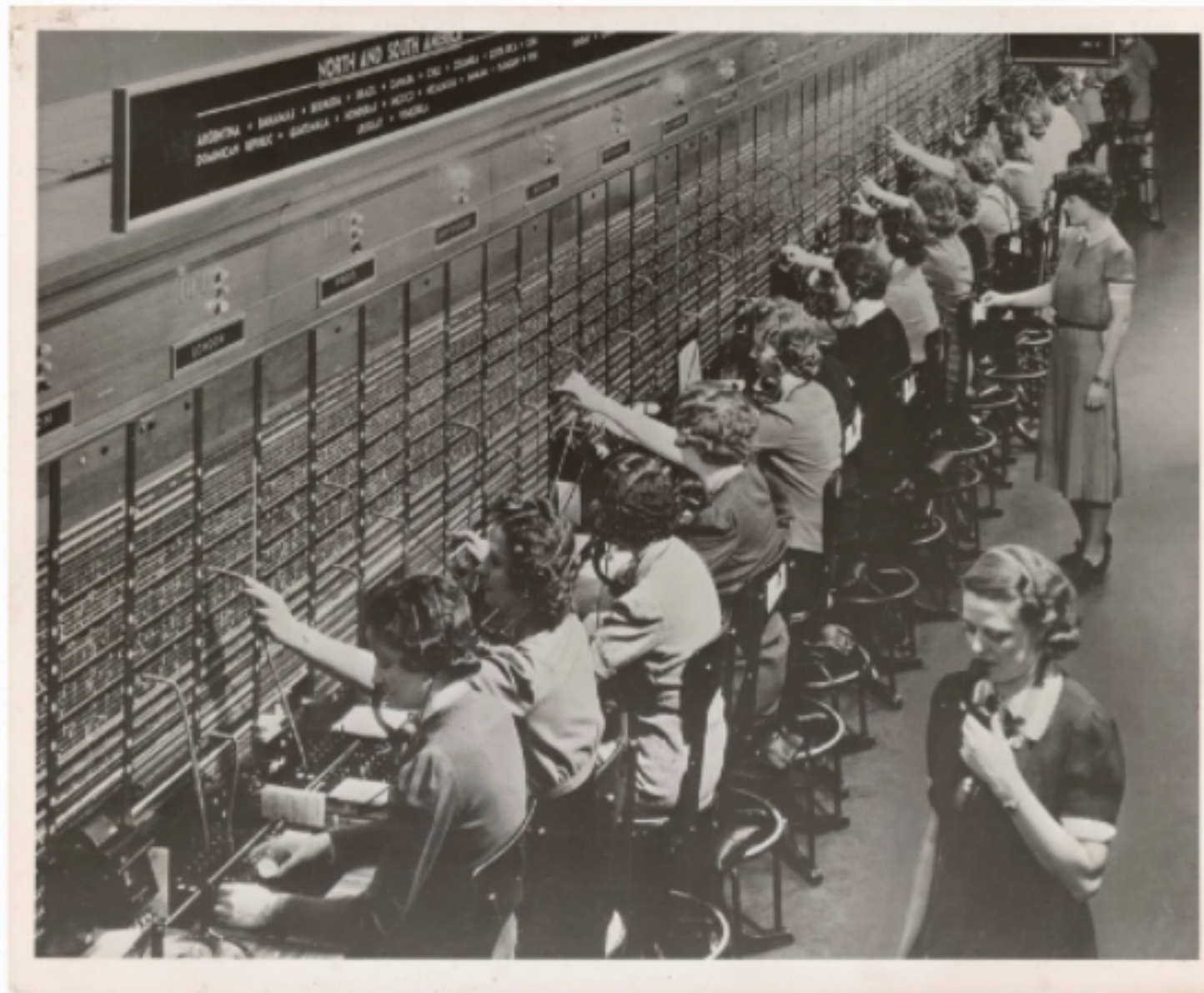
A large Bell System international switchboard in 1943
