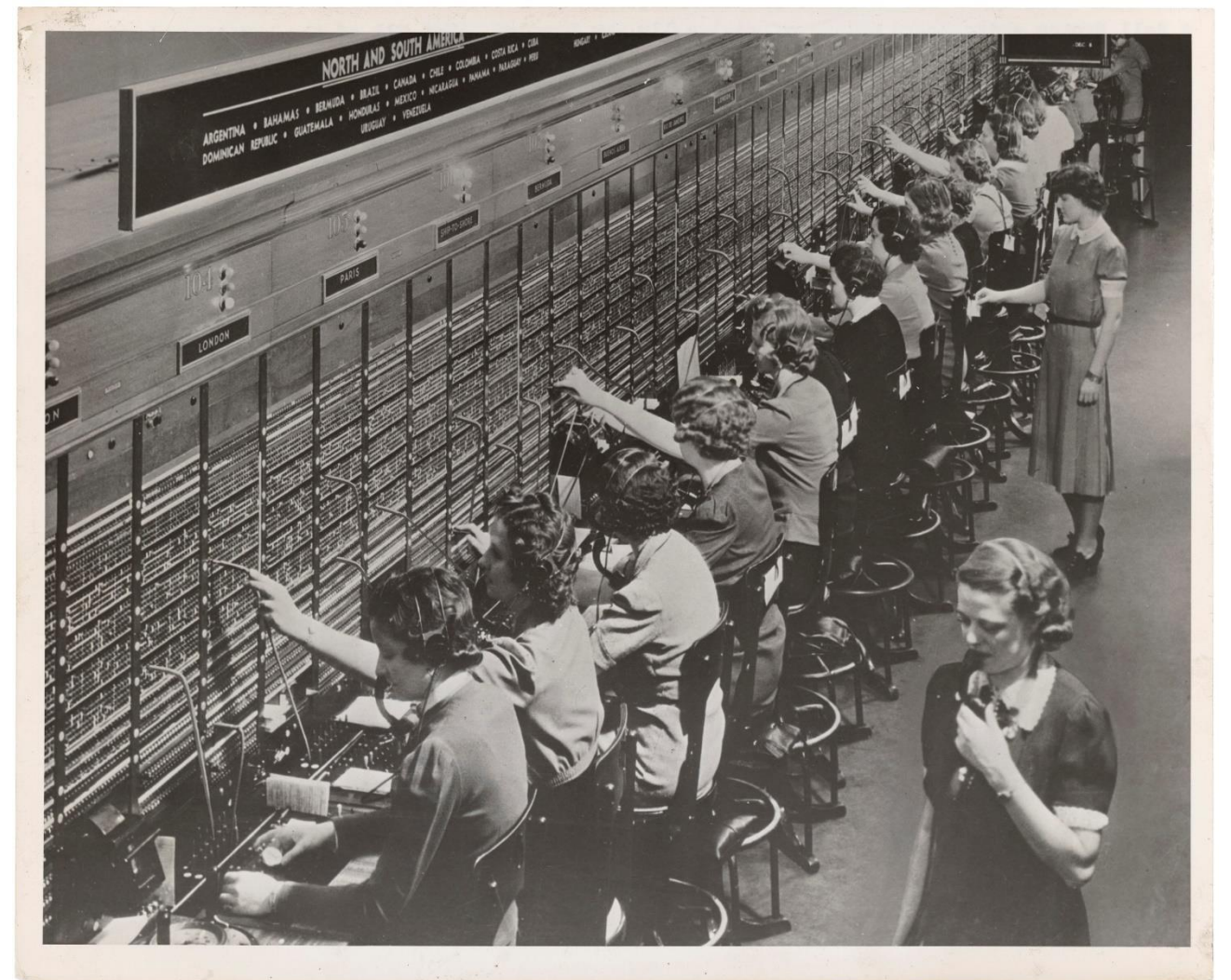
A large Bell System international switchboard in 1943
